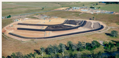
CEDAR GROVE WASTE WATER TREATMENT PLANT TIMING: 2019 - 2019 | VALUE: $4M
