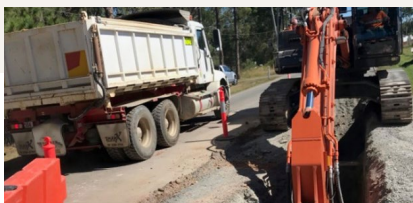
ANDREW ROAD, GREENBANK - DEEP GRAVITY SEWER SYSTEM TIMING: 2019 - 2019 | VALUE: $4M
