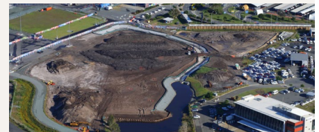
GROUND TRANSPORT INFRASTRUCTURE TIMING: 2017 - 2018 | VALUE: 9.6M
