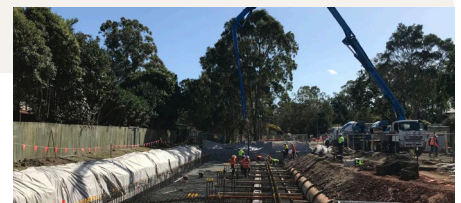
PRIESTDALE RD, ROCHEDALE - SEWER & STORMWATER INFRASTRUCTURE UPGRADES TIMING: 2020 - 2020 | VALUE: $2.3M
