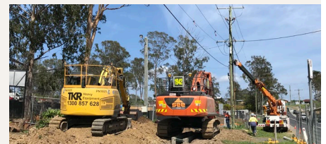
EAST STREET SEWER PUMP STATION AND RISING MAIN TIMING: 2020-2020 | VALUE: $2.5M
