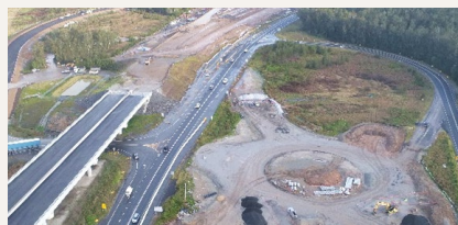
PACIFIC HIGHWAY UPGRADE WOOLGOOLGA TO BALLINA EARTHWORKS PACKAGE 2 TIMING: 2019 - 2020 | VALUE: $30M
